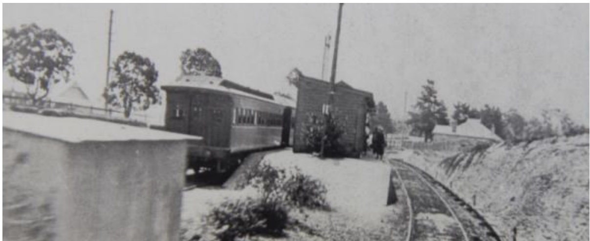
Baulkham Hills island platform 1923
