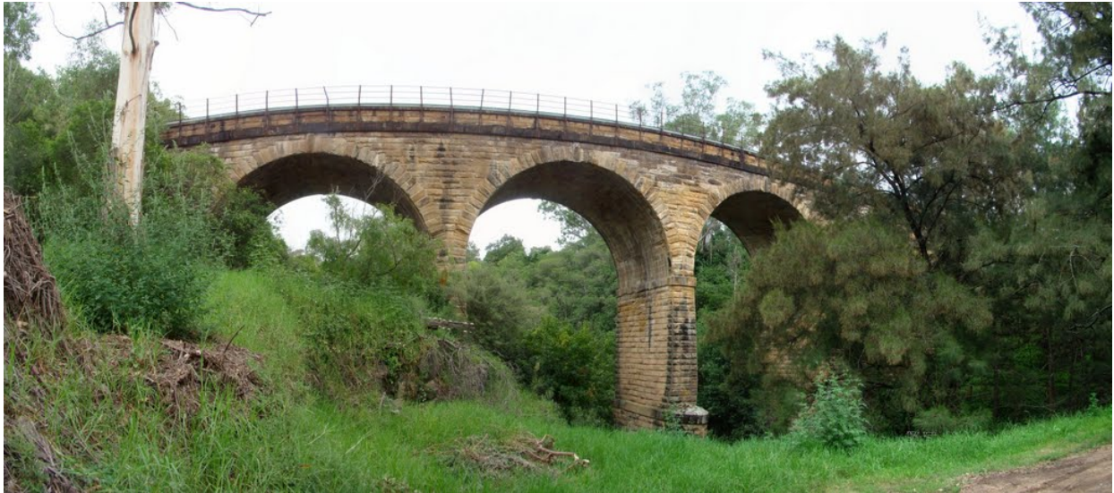
Picton viaduct over Stone quarry creek
